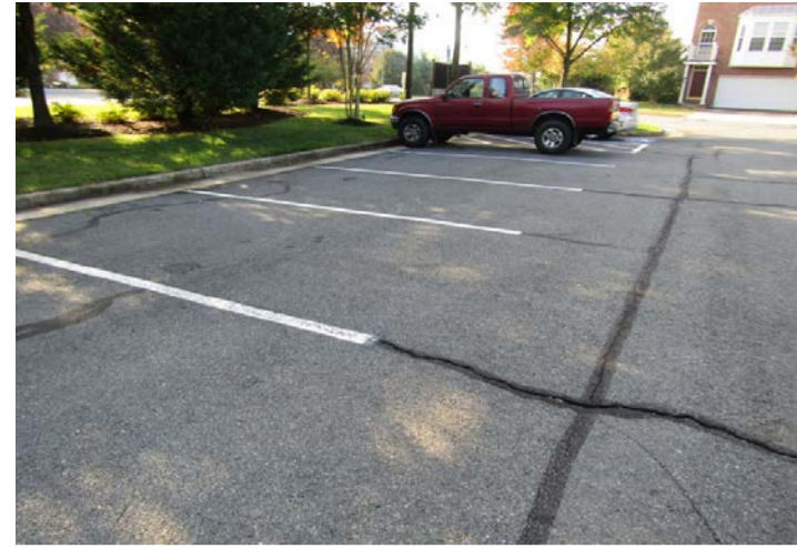
asphalt pavement at pool house parking
