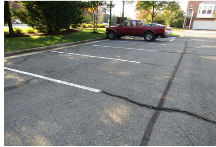
asphalt pavement at pool house parking
