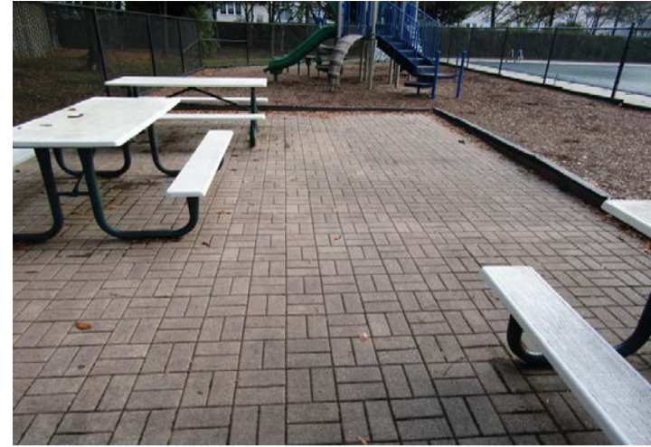
basketweave pattern dry set masonry pavers
