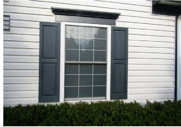
vinyl frame, dual pane glass, double hung window with decorative muntins
