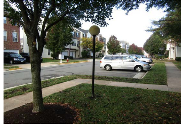
metal light pole with globe light fixture
