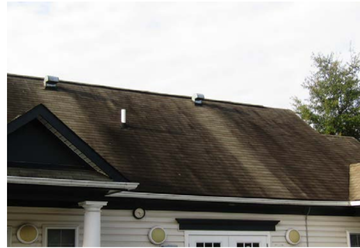
weathered shingles
