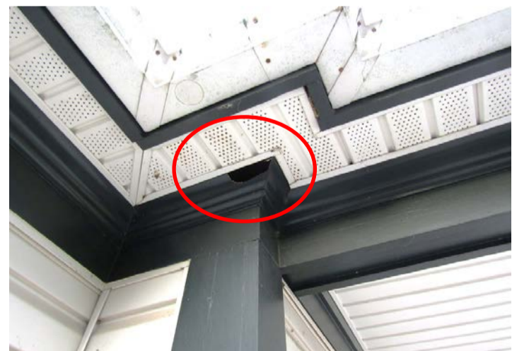
void in trim allows for insects/pests
