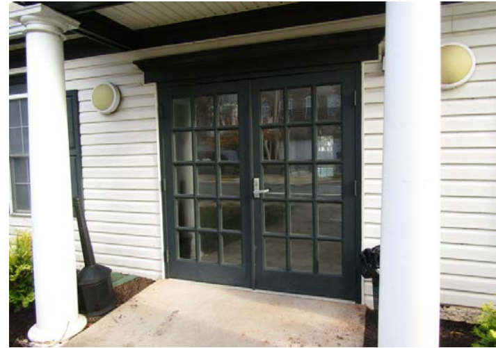
wood entrance doors
