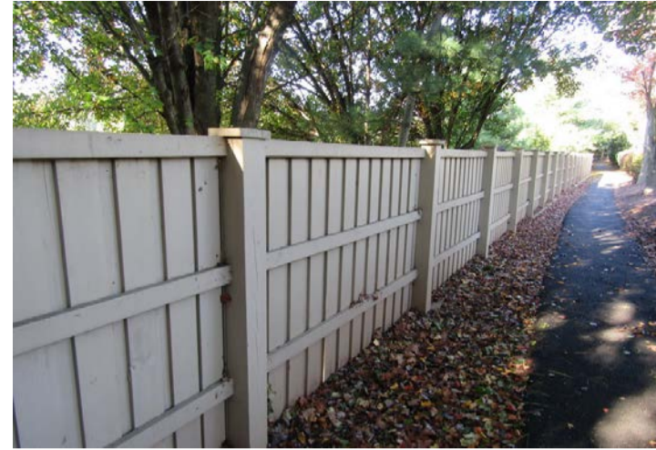
shadowbox wood fence at Southern Oaks Terrace
