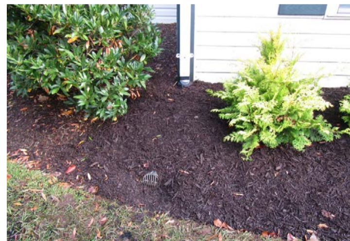
downspout discharge
