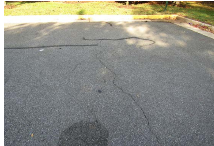
open cracks
