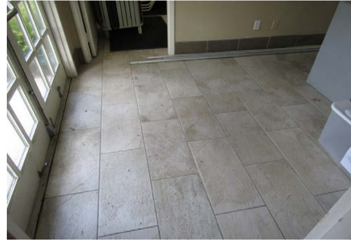
12 inch by 24 inch tile typical of the pool house interior with tile transition at floor to wall
