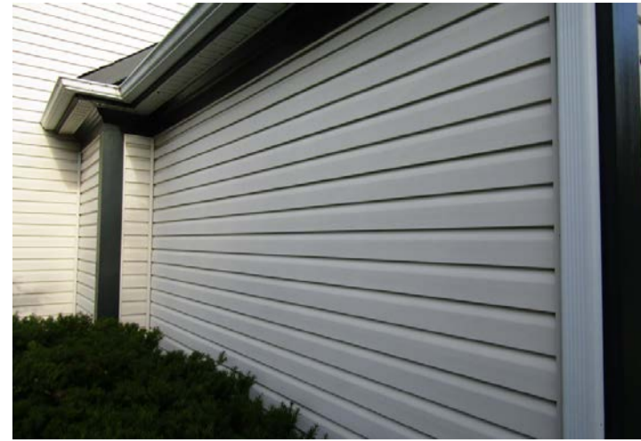
vinyl siding with Dutch lap profile
