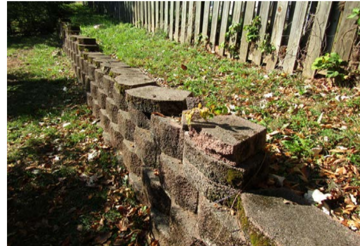
block deterioration
