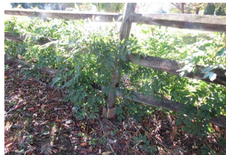
leaning section and repair to post rot
