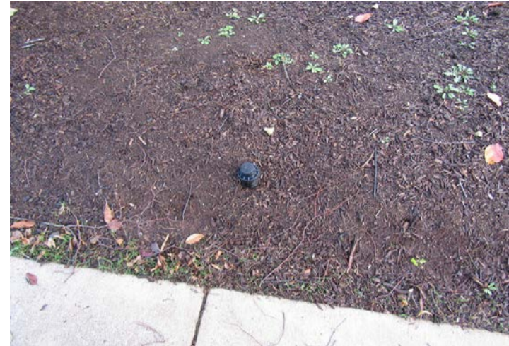
irrigation system head
