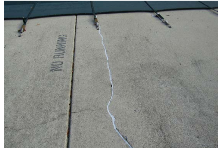
repaired crack
