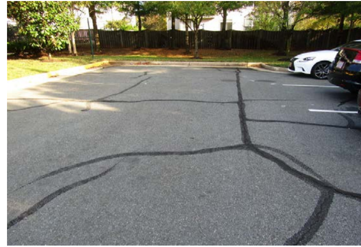
crack repairs at parking area
