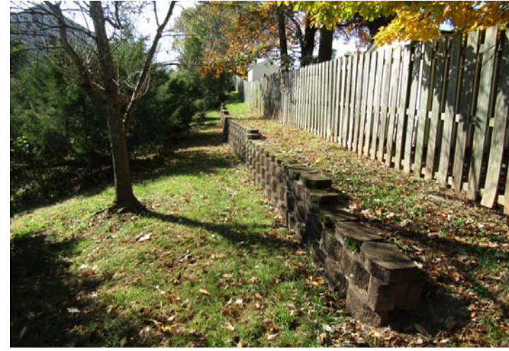
masonry retaining wall
