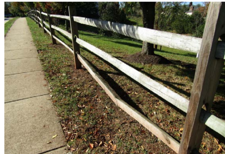
isolated picket damage at Backwater
