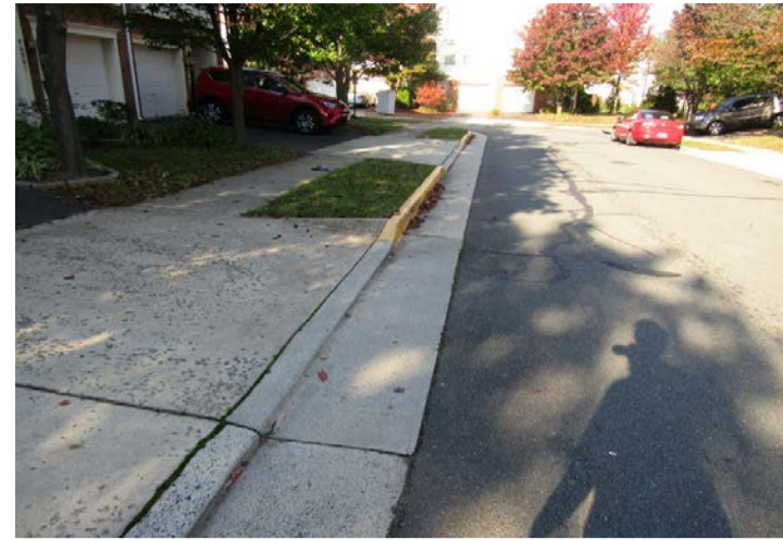
30 inch concrete curbs and gutters
