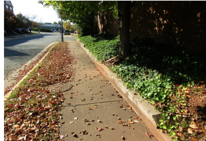
leaning retaining wall
