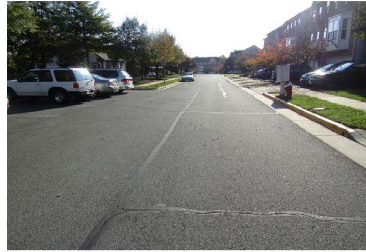
asphalt pavement at streets and parking areas
