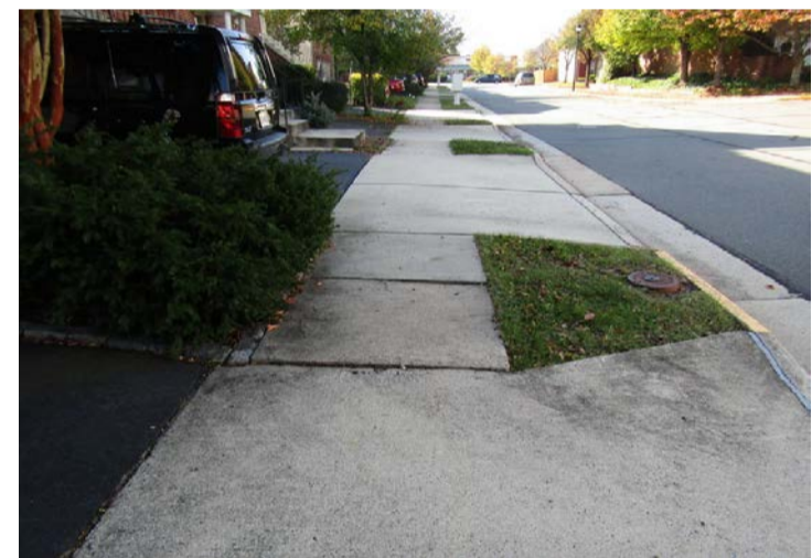
concrete aprons, sidewalks, curbs and gutters
