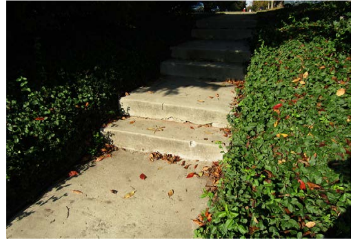
concrete sidewalks and steps
