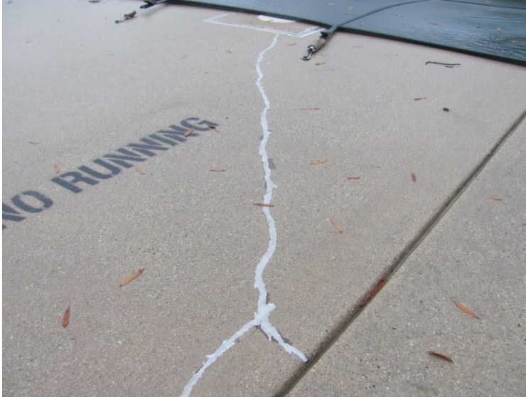
Concrete pool deck crack repairs
