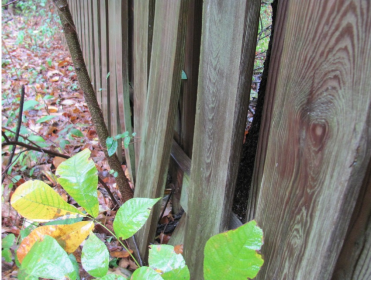
Shadowbox wood stockade fence board warp
