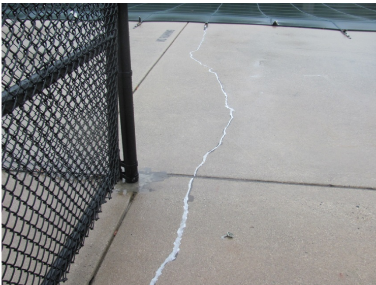
Concrete pool deck crack repairs
