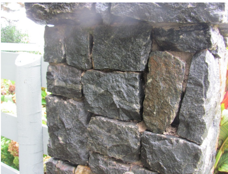
Masonry pillar accents at entrance monument signage
