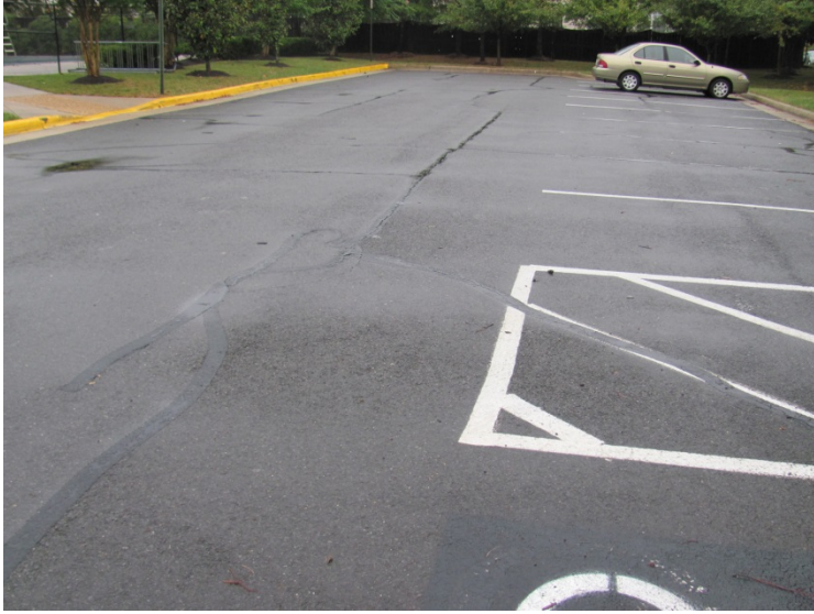
Asphalt pavement pool parking area
