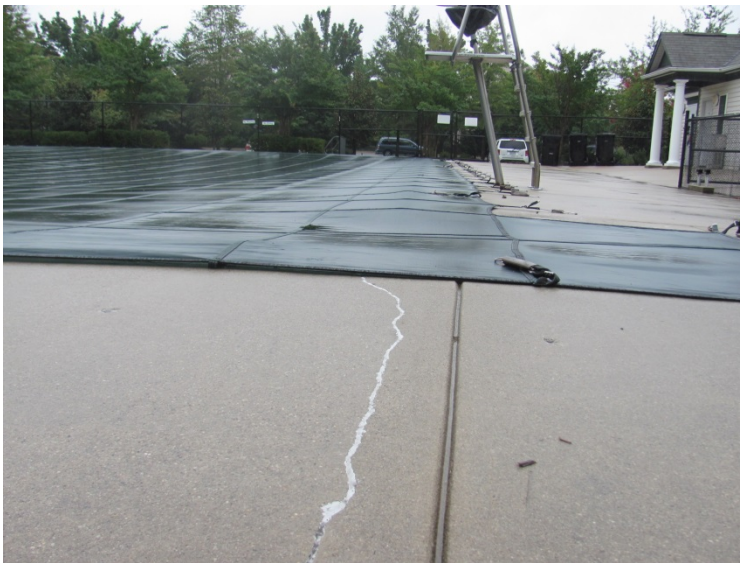
Concrete pool deck crack repairs
