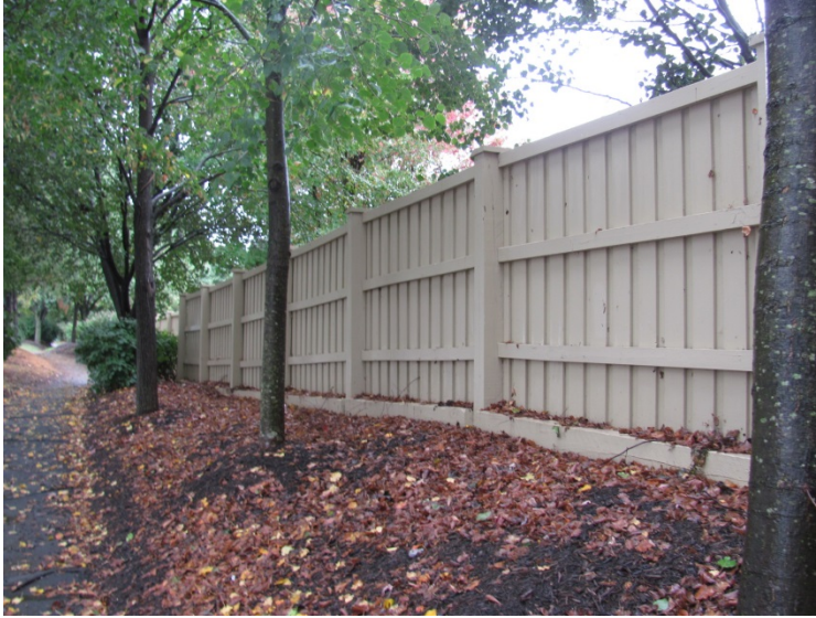
Painted fence along asphalt pavement walking path
