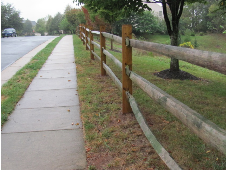
Wood split rail fence at retention basin
