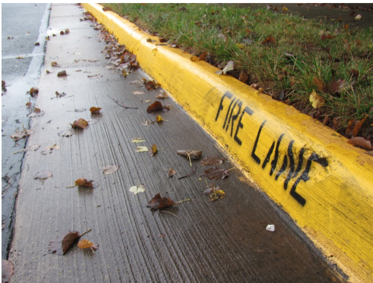
Townhome concrete curb and gutter
