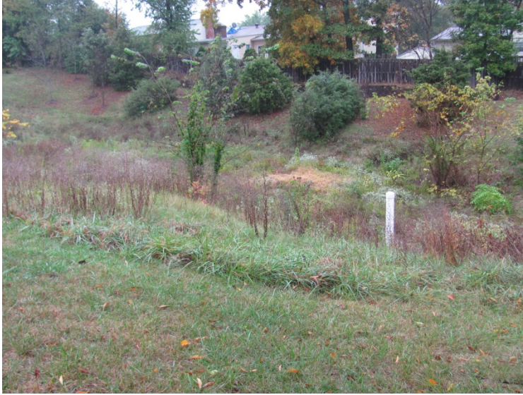
Retention basin near Backwater Drive
