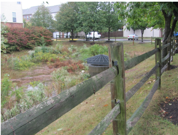
Wood split rail fence at retention basin
