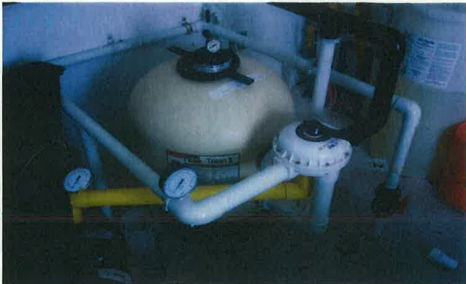
PHOTOGRAPH 10: Sand Filter for Wading Pool
