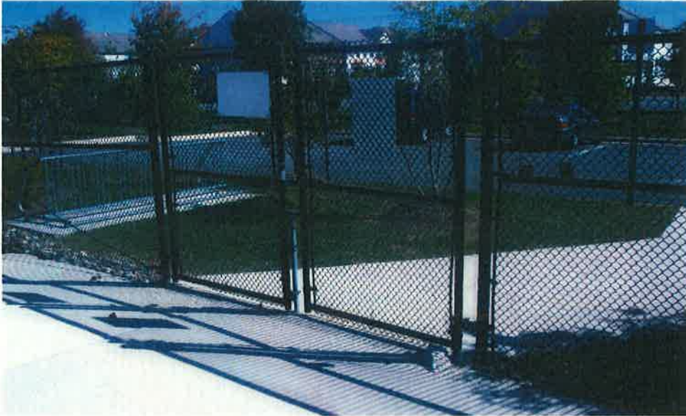
PHOTOGRAPH 1: Vinyl-Covered Chain-Link Fencing at Pool Area
