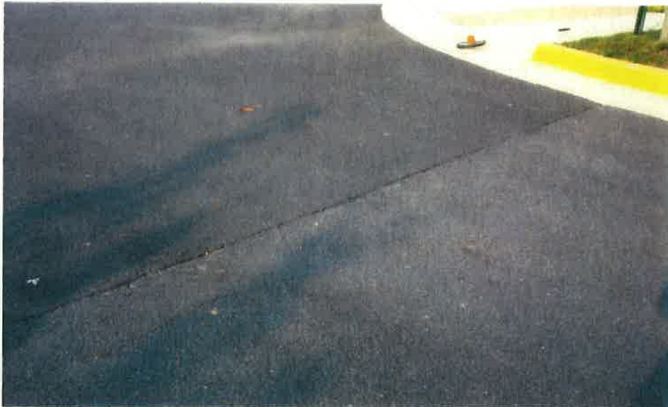
PHOTOGRAPH 25: Example of Minor Asphalt Cracking at Joints
