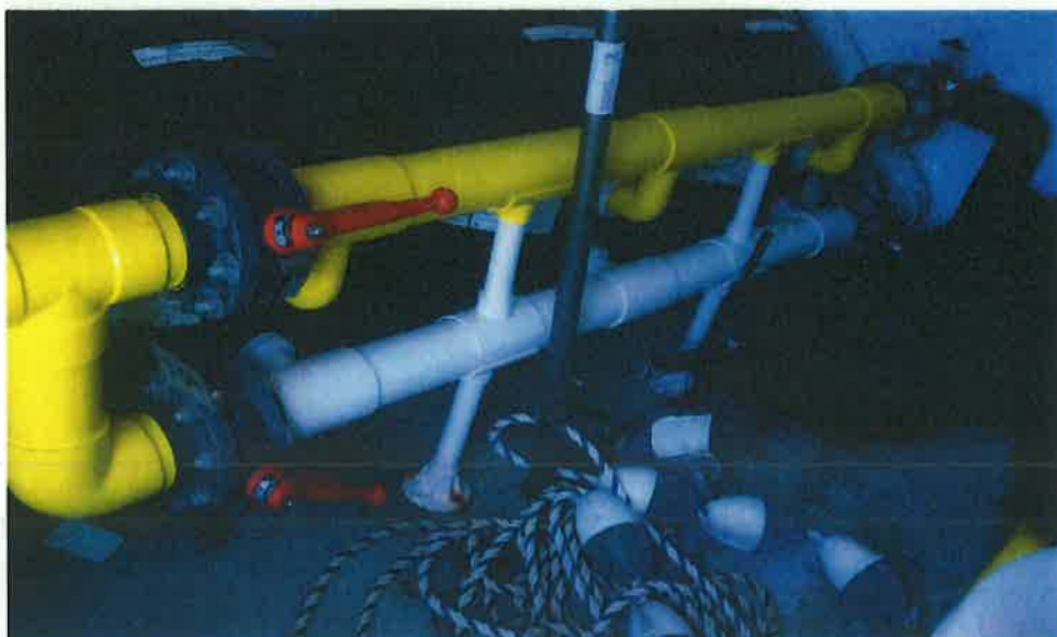
PHOTOGRAPH 9: Sand Filters and Valve System for Main Pool
