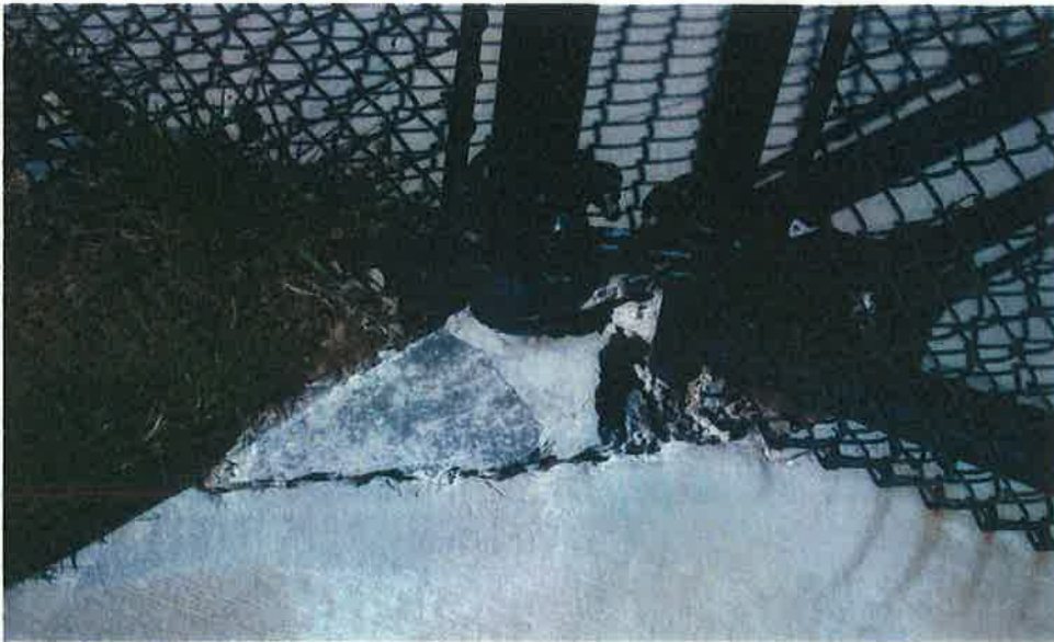
PHOTOGRAPH 13: Severe Deterioration of Concrete in Pool Area
